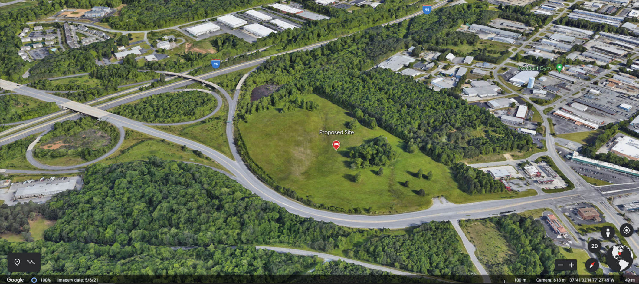
HANOVER HOSPITAL OVERVIEW
