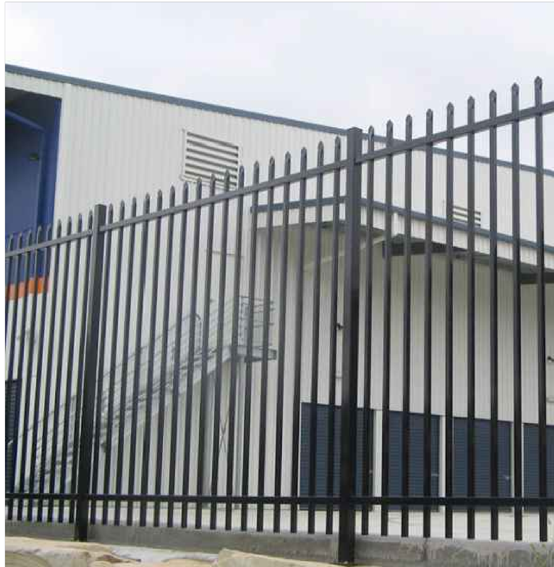
EXAMPLE PERIMETER/SECURITY FENCING
